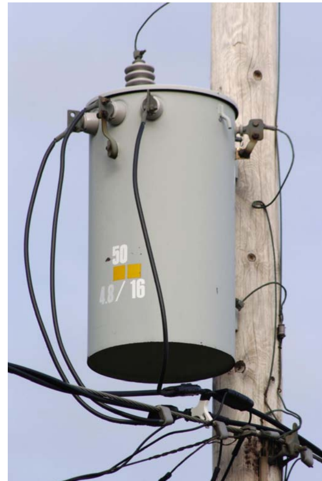
Distribution Transformer
